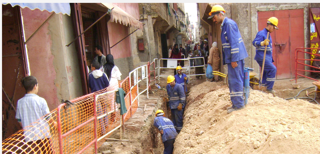
Workers digging a trench for a water pipe (Lydec, 2016)
